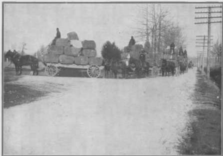
FIG. 2.—JUNCTION OF CHESTER LEVEE AND BEMIS ROADS, NEAR JACKSON, TENN.
