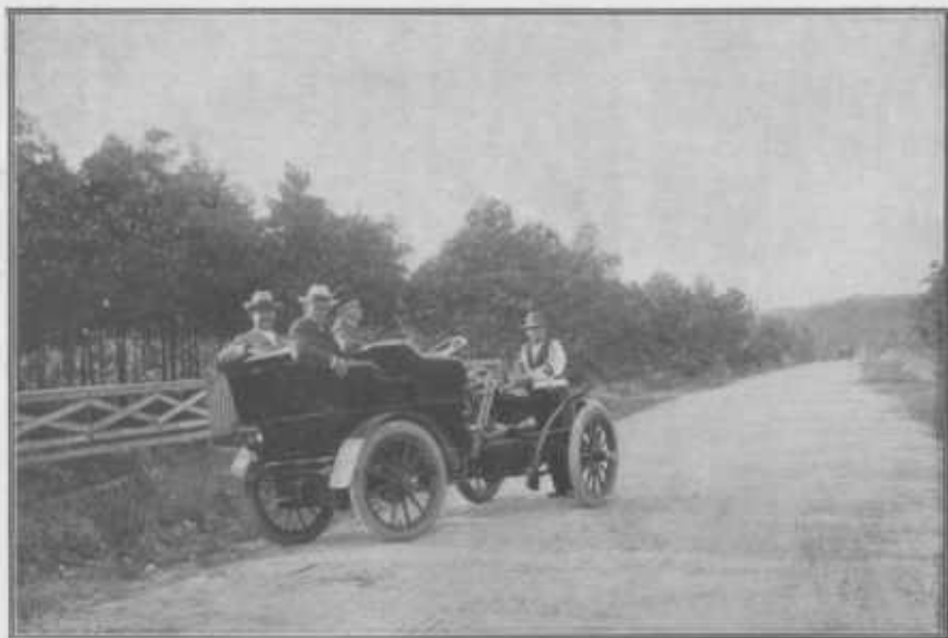
FIG. 1.—THE JOPLIN, MO. SPECIAL ROAD DISTRICT COMMITTEE INSPECTING THE FINE ROADS CONSTRUCTED OF MINING SLAG UNDER THEIR SUPERVISION.
