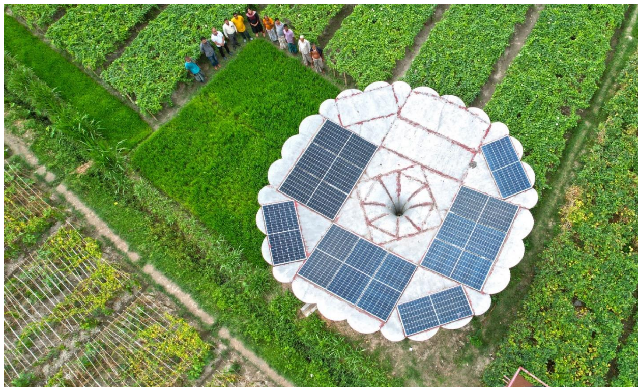
A SoLAR installation with rainwater harvesting facility ( photo : Waresul Haque, NGO-Forum)
