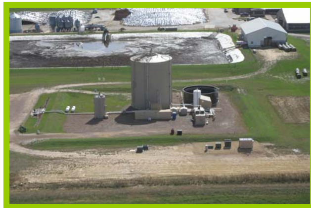
Waste-to- Energy Systems (Manure Digesters)
