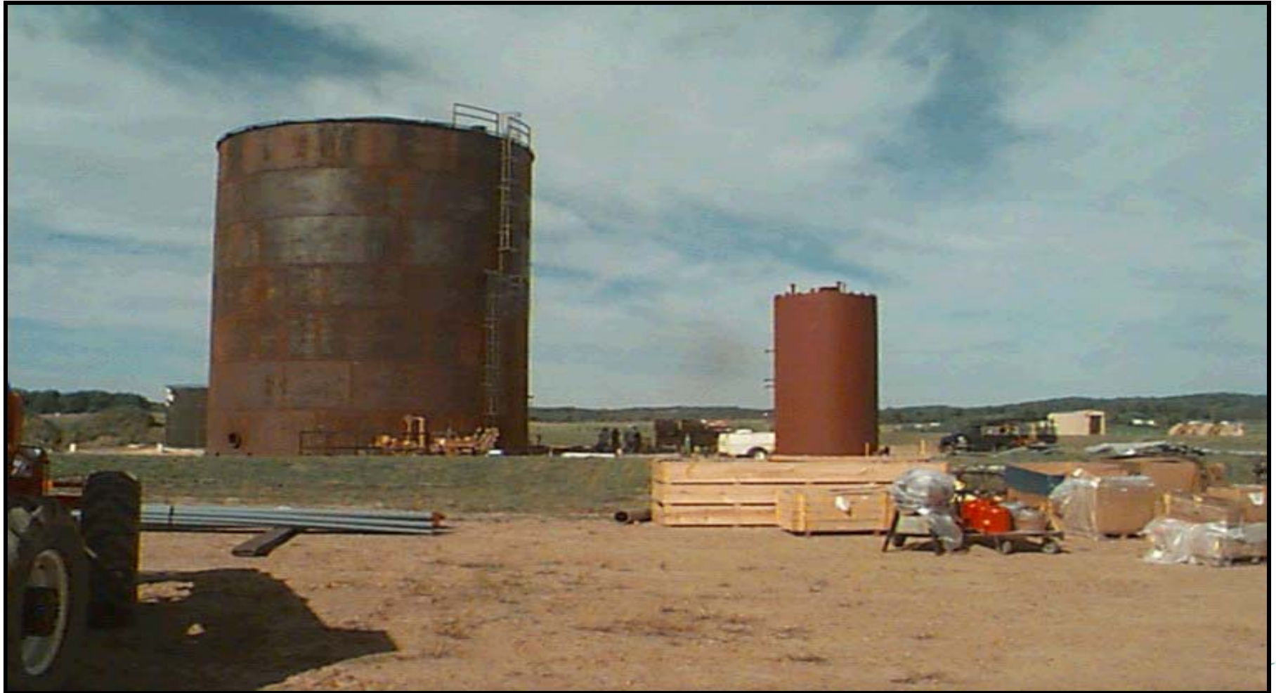
Digester tank and substrate tank
