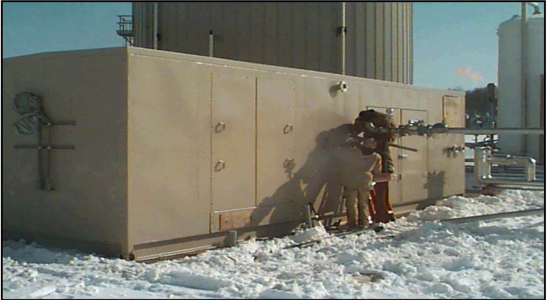
Arrival of engine / generator set
