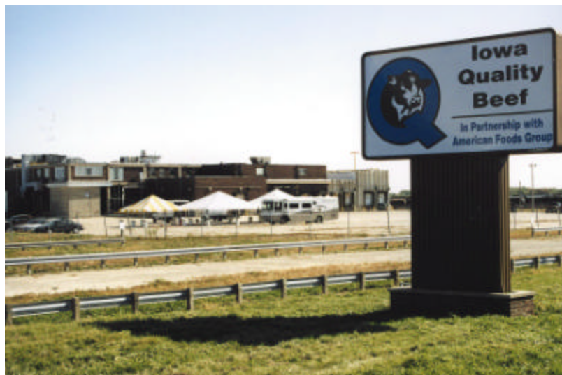
The Iowa Quality Beef Supply Cooperative harvest facility will open this spring in Tama, Iowa. At full capacity, about 1,200 cattle will be processed daily.
