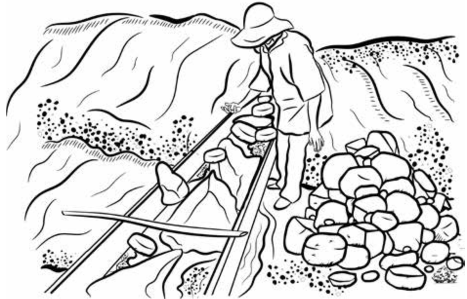
Construction of stone boulder embankment dam across a stream
