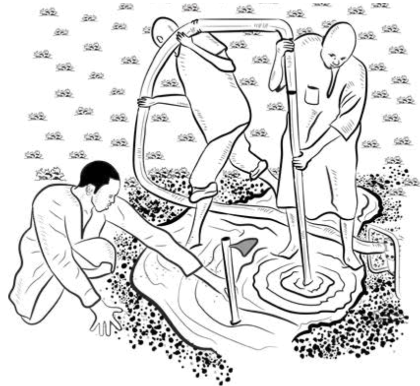
Step 4: Drilling tube well by jetting from water pump pressure
