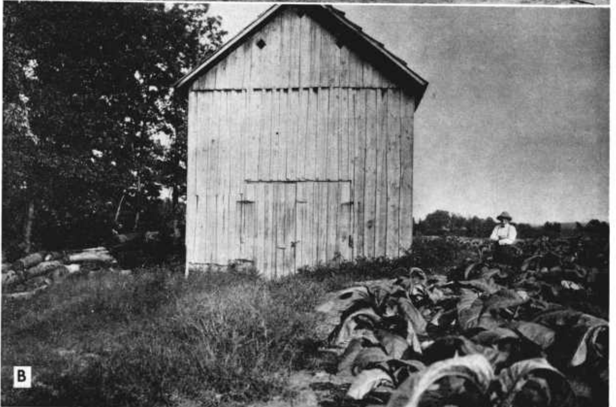
FIGURE 21.—Type of barn used in fire-cured districts of Kentucky and Tennessee: A , Fire-cured leaf hanging in barn with remnants of fire on the ground; B , exterior view of the barn.
