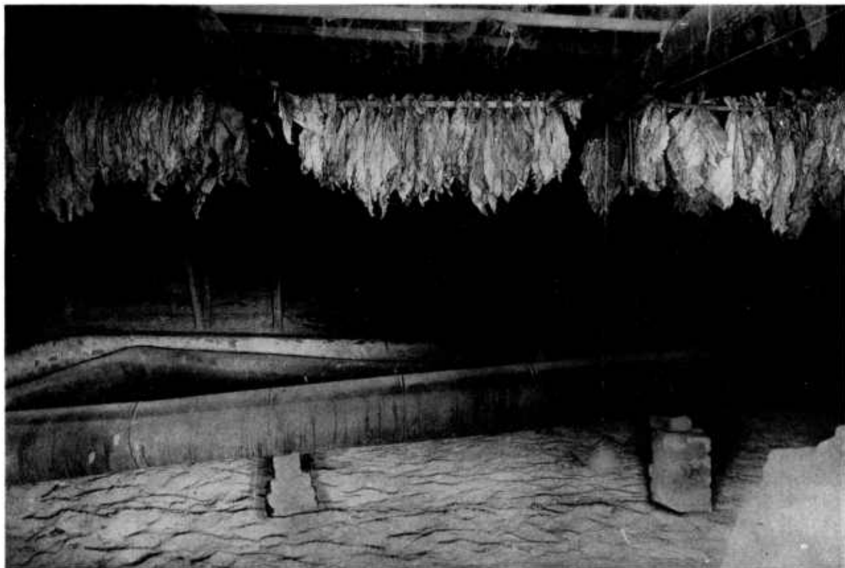
FIGURE 19.—Flue-curing tobacco barn interior, showing flues and cured leaf just before its removal after curing.
