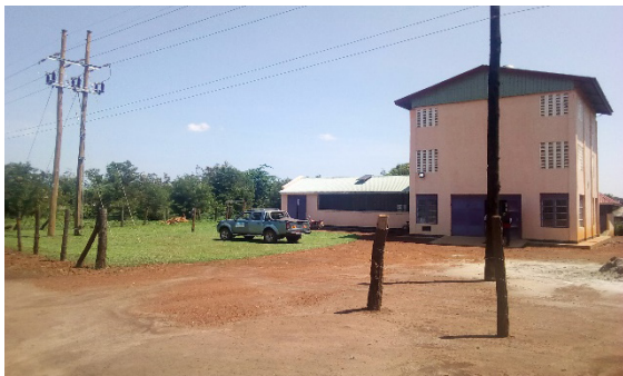
Plate 1: Inaccessible power to Factory in Apac
