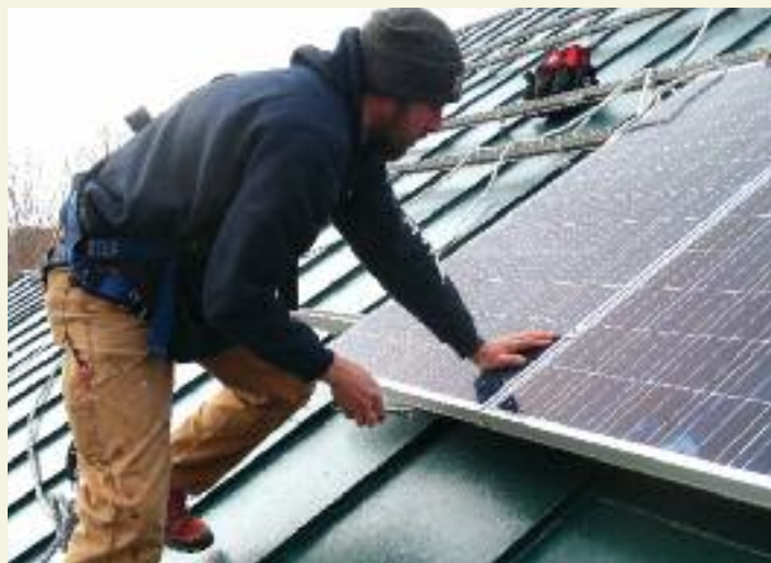
An Insource Renewables crew installs rooftop solar panels. The business is in the process of converting to a worker-owned co-op. Photo courtesy Insource Renewables
