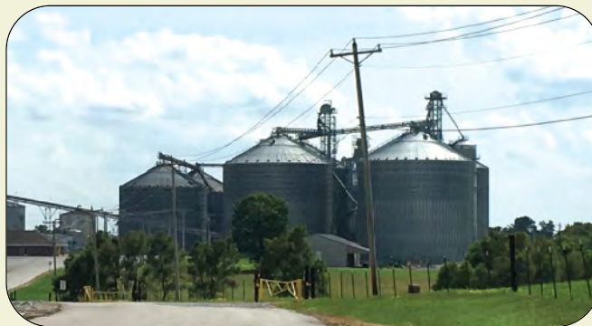
This facility is operated by Hopkinsville Elevator.
