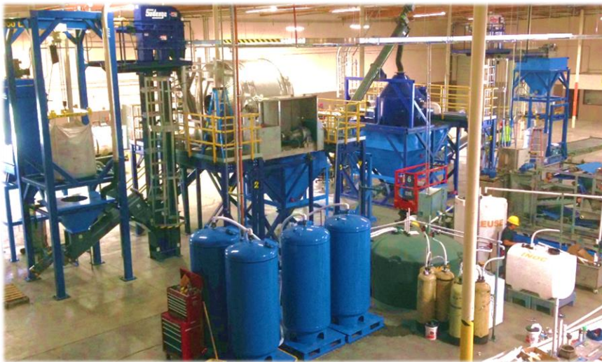
40,000 yd 3 capacity in Camarillo, CA
