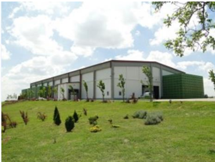
Figure 1. The exterior of ULO cold storage
