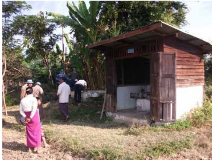
FIGURE A2. Pump house for a community irrigation well 4/1 (the stilling tank before distribution is evident to the left of the image).
