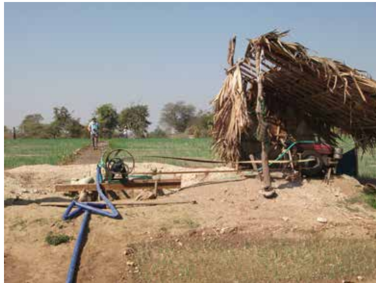
FIGURE A5. The newly constructed deep well which pumps water that is manually spread across the first crop of onions.
