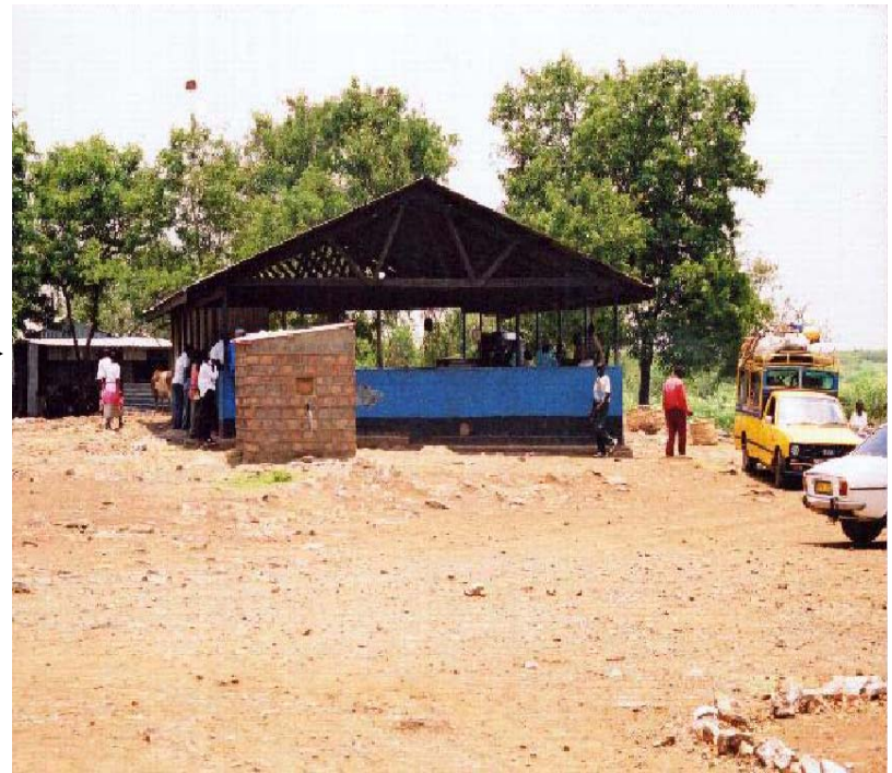
Landing facility with pit latrine, wall, roof
