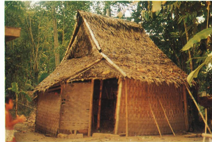
Photograph 1.5.3 A closed-sided cattle house with bamboo-plaited walls in Betung II- B, South Sumatera.
